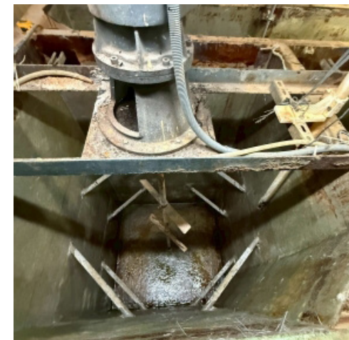
Stage 2 Wastewater Treatment Plant Motor Replacement and Aeration Tank Upgrade Project (FRP Lining and Motor Replacement)
