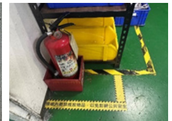
Fire Safety Equipment Enhanced Warning Lines
