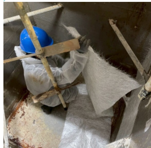
Stage 2 Wastewater Treatment Plant Motor Replacement and Aeration Tank Upgrade Project (FRP Lining and Motor Replacement)
