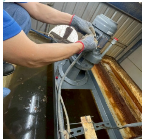
Stage 2 Wastewater Treatment Plant Motor Replacement and Aeration Tank Upgrade Project (FRP Lining and Motor Replacement)
