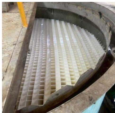
Stage 1 Wastewater Chemical Treatment System Reinforcement Project – Sedimentation Tank Rehabilitation (FRP Lining and Filter Media Replacement)
