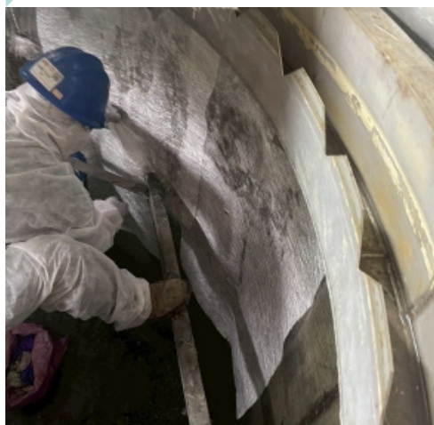
Stage 1 Wastewater Chemical Treatment System Reinforcement Project – Sedimentation Tank Rehabilitation (FRP Lining and Filter Media Replacement)
