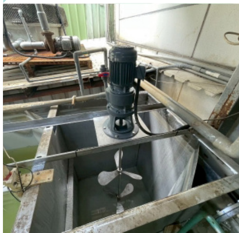
Stage 1 Wastewater Chemical Treatment System Reinforcement Project – Sedimentation Tank Rehabilitation (FRP Lining and Filter Media Replacement)
