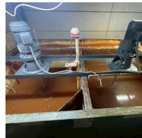
Stage 2 Wastewater Treatment Plant Motor Replacement and Aeration Tank Upgrade Project (FRP Lining and Motor Replacement)
